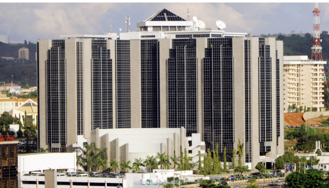
Cryptic: The Central Bank of Nigeria HQ in Abuja
