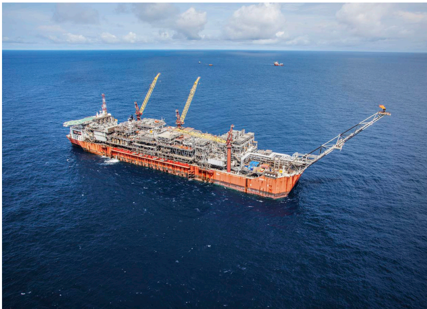
Fuel's errand: Shell's Bonga oil plant in the Gulf of Guinea. A court has ruled Shell must cut emissions in the Netherlands by 45% in nine years. Photo: Shell, 2015
