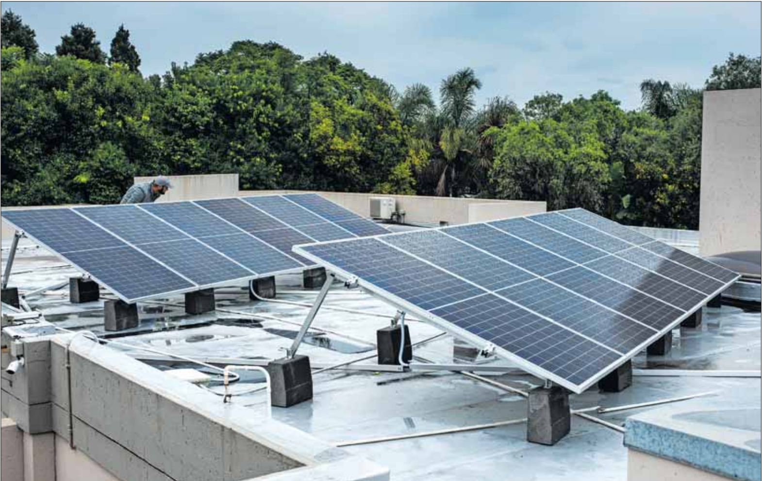
Security: Make sure your solar panels are securely bolted on the roof to discourage theft. Photo: Waldo Swiegers/Getty Images
