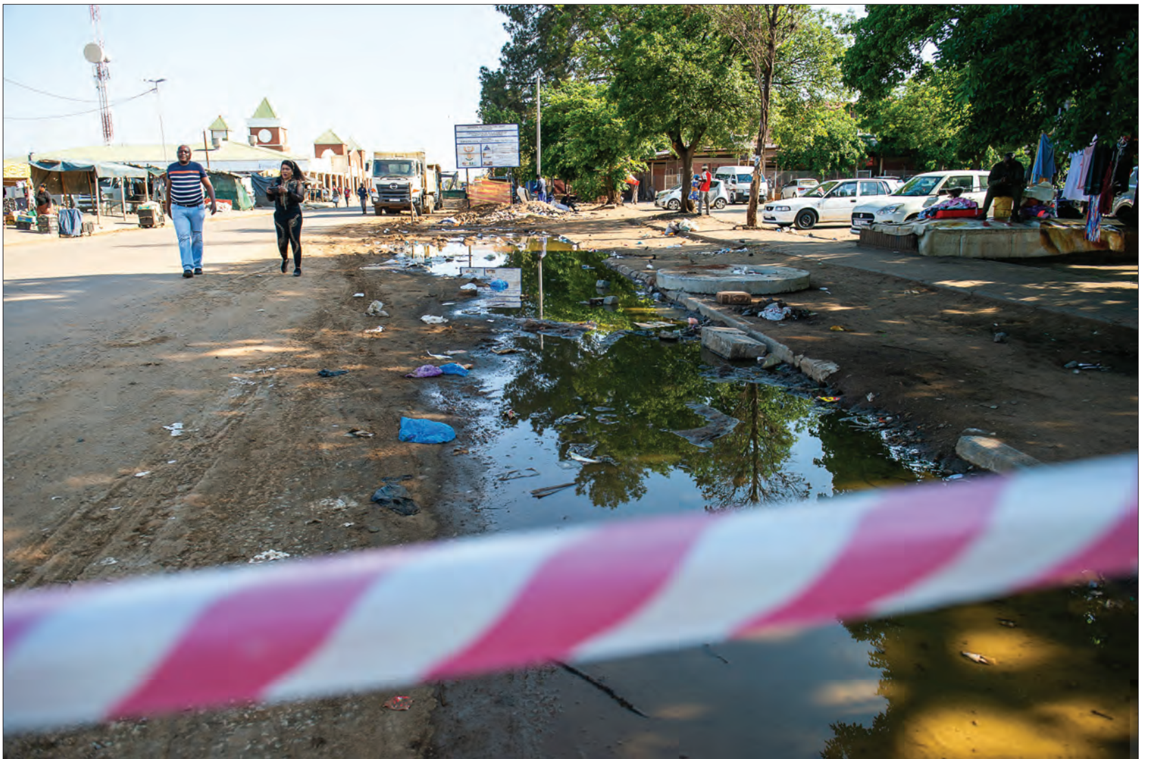
Dysfunctional: Infrastructure failure and lack of repair and upgrade, seen on a road at a taxi rank in Emfuleni. The municipality is in a complete state of failure. Photo: Delwyn Verasamy
